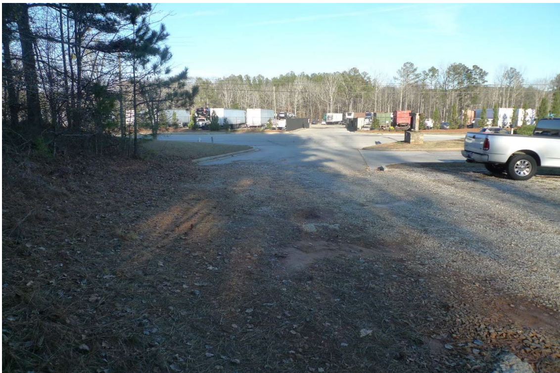
View of Subject Project access driveway facing east from Cedars Road.
